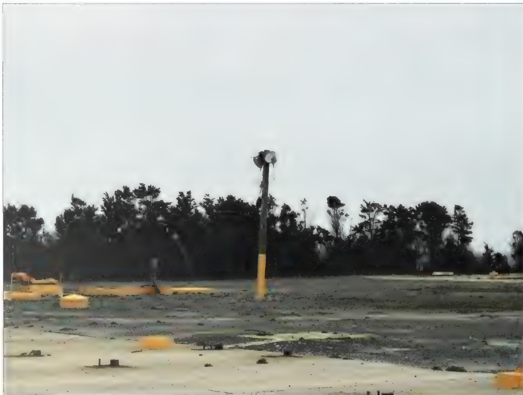
Figure 3.72. Spotlights, NIKE launch site. In the Missile Magazine area a single, round, wood pole stands near the Section B magazine (427). The first eight to ten feet of the pole are painted yellow and two spotlights with parabolic metal hoods are mounted at the top of the pole (Olmsted Center, April 2008).
